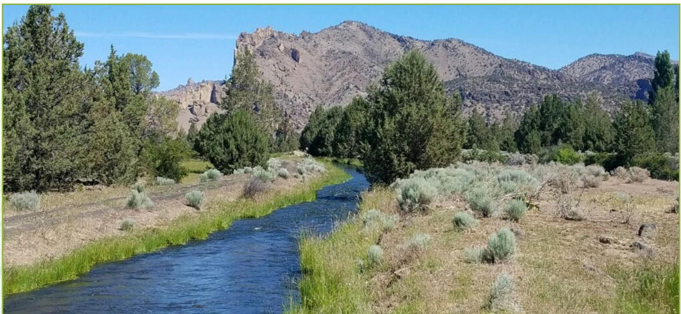
Central Oregon Irrigation District open canal. Photo credit: Oregon DEQ
