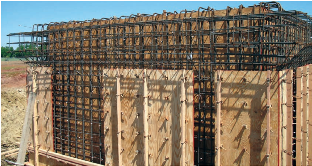
Washington County Rural Water District #3- Rebar for High Service Pump Station.
