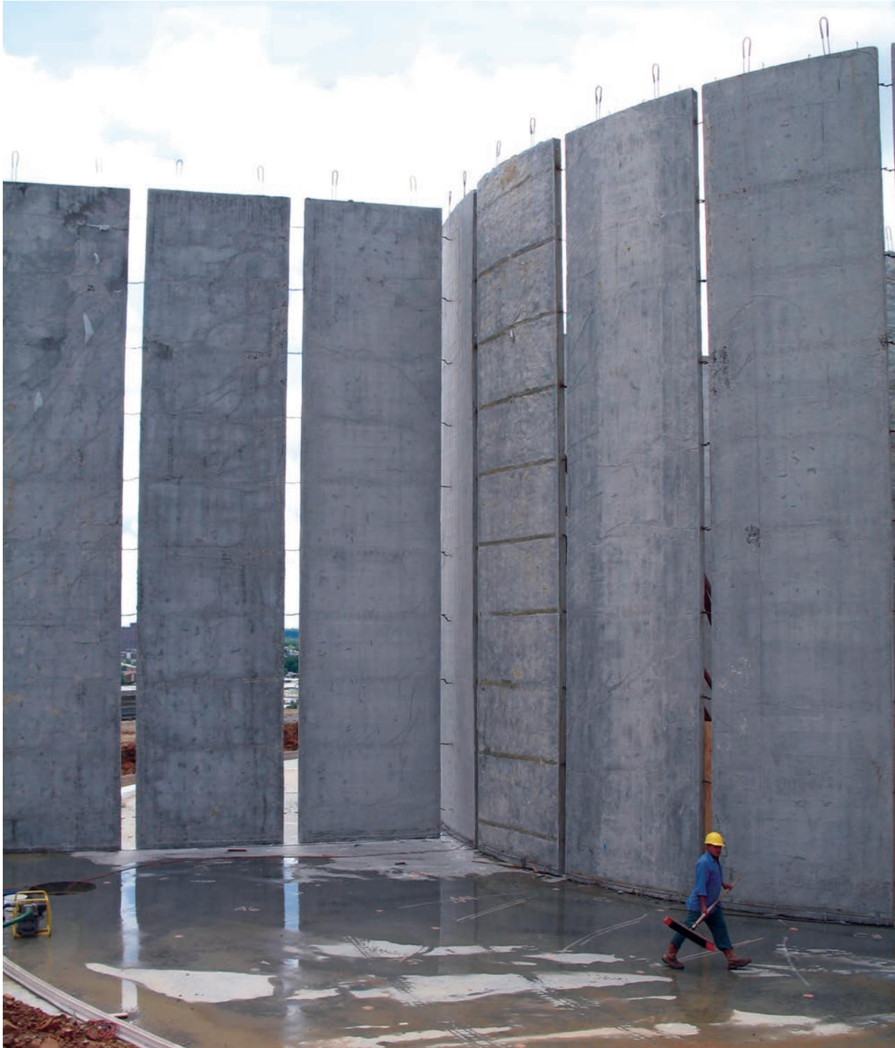
Bartlesville-Construction of interior wall for a 4 million gallon storage tank.
