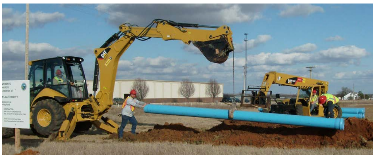
Newcastle-Construction of water line
