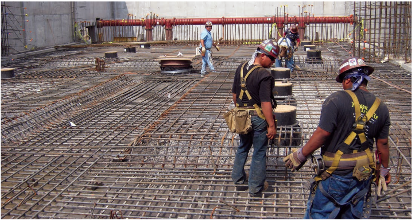
Muskogee-Concrete and rebar for construction of Super Pulsators.
