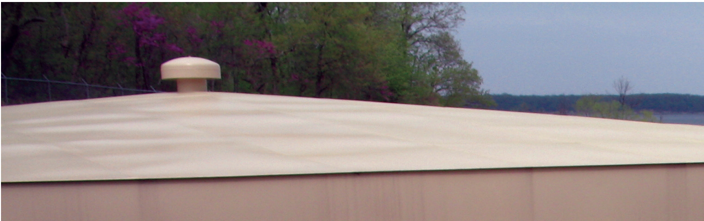
Rogers Rural Water District # 3-Construction of clearwell near Lake Oologah.
