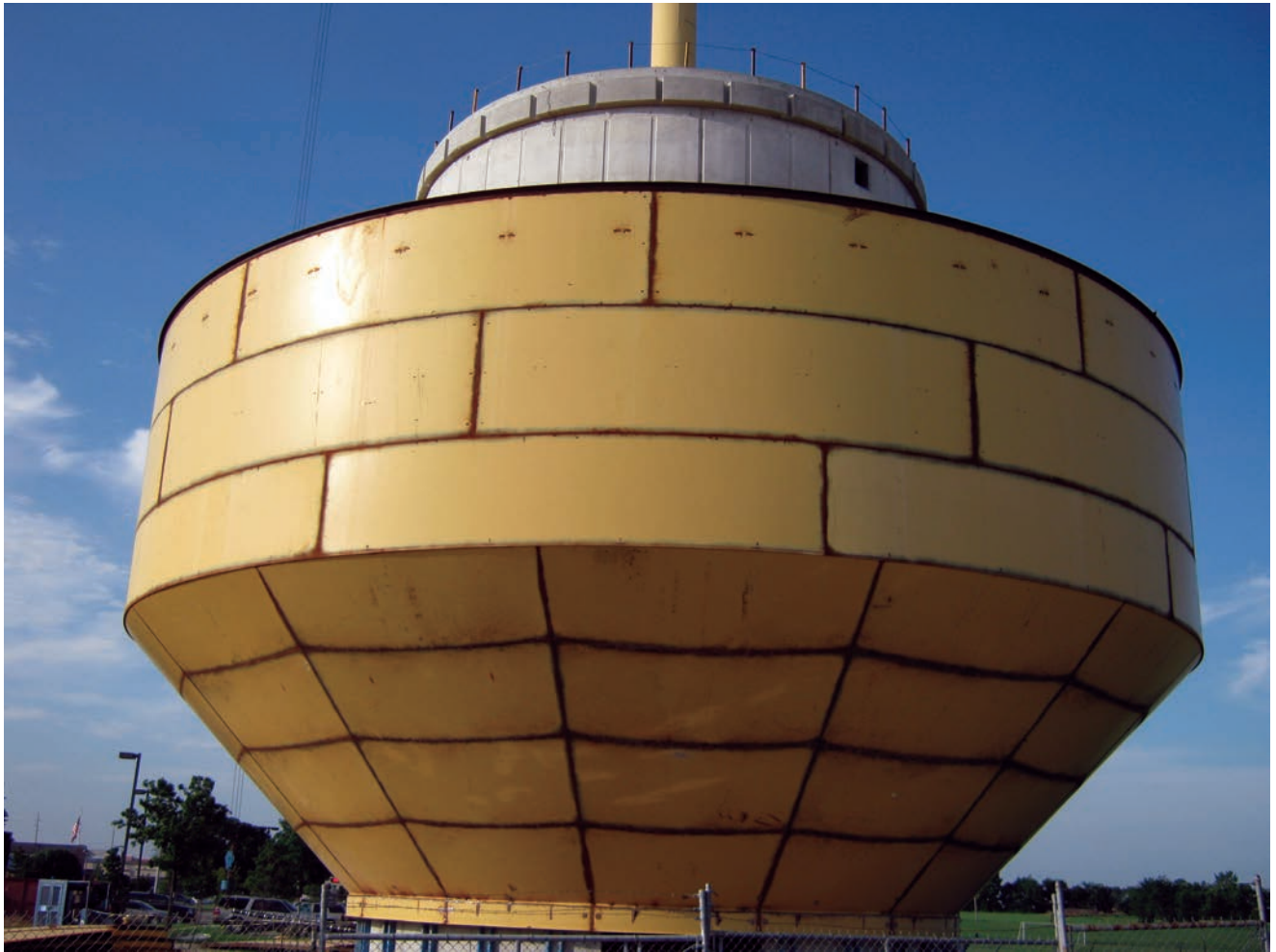
Ardmore-Construction of 2 million gallon elevated storage tank.
