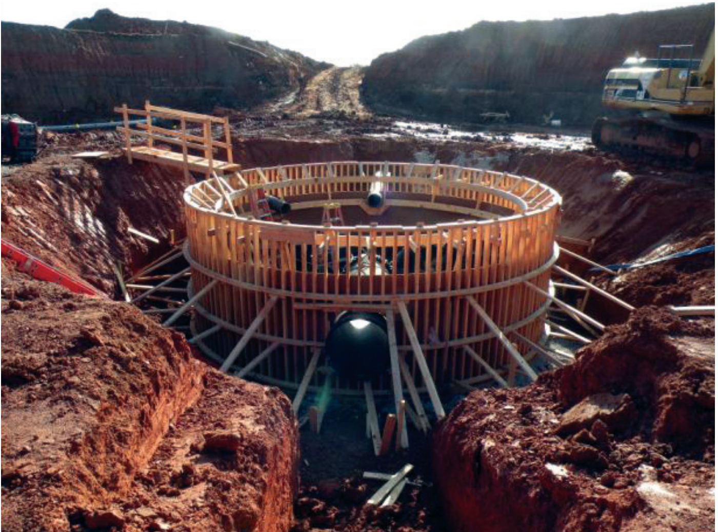
Norman-Construction of 10 MGD solids contact clarifier.
