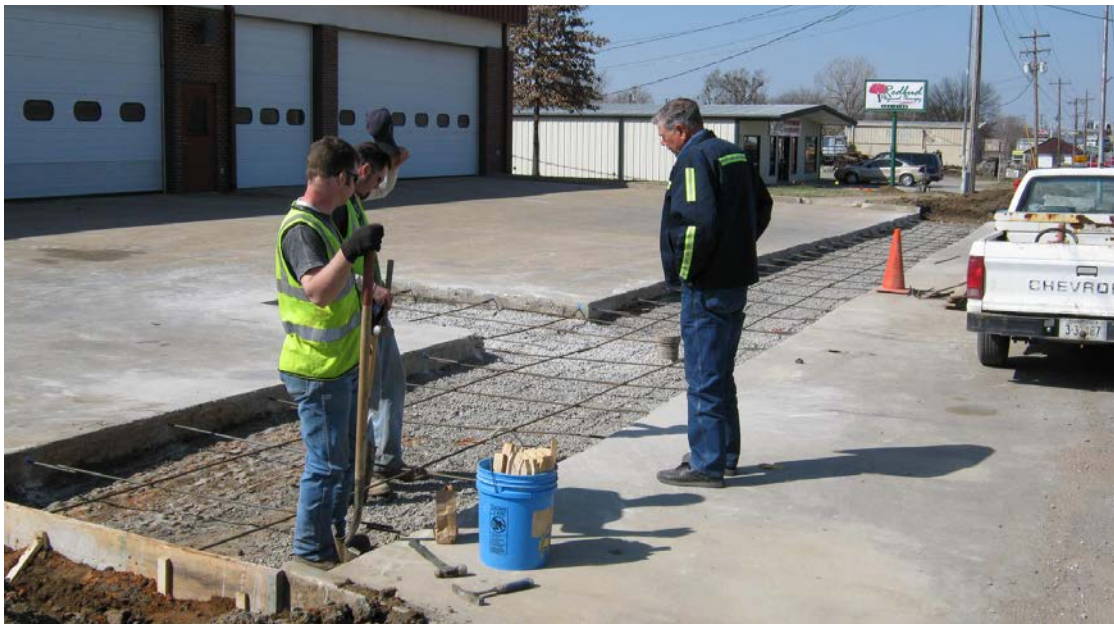
Wagoner-Pavement repair being completed after line replacement.
