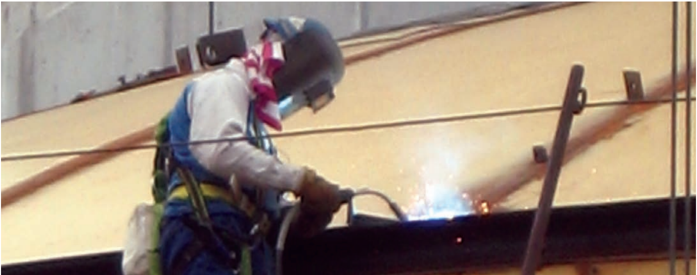
Ardmore-Construction of 2 million gallon elevated storage tank.
