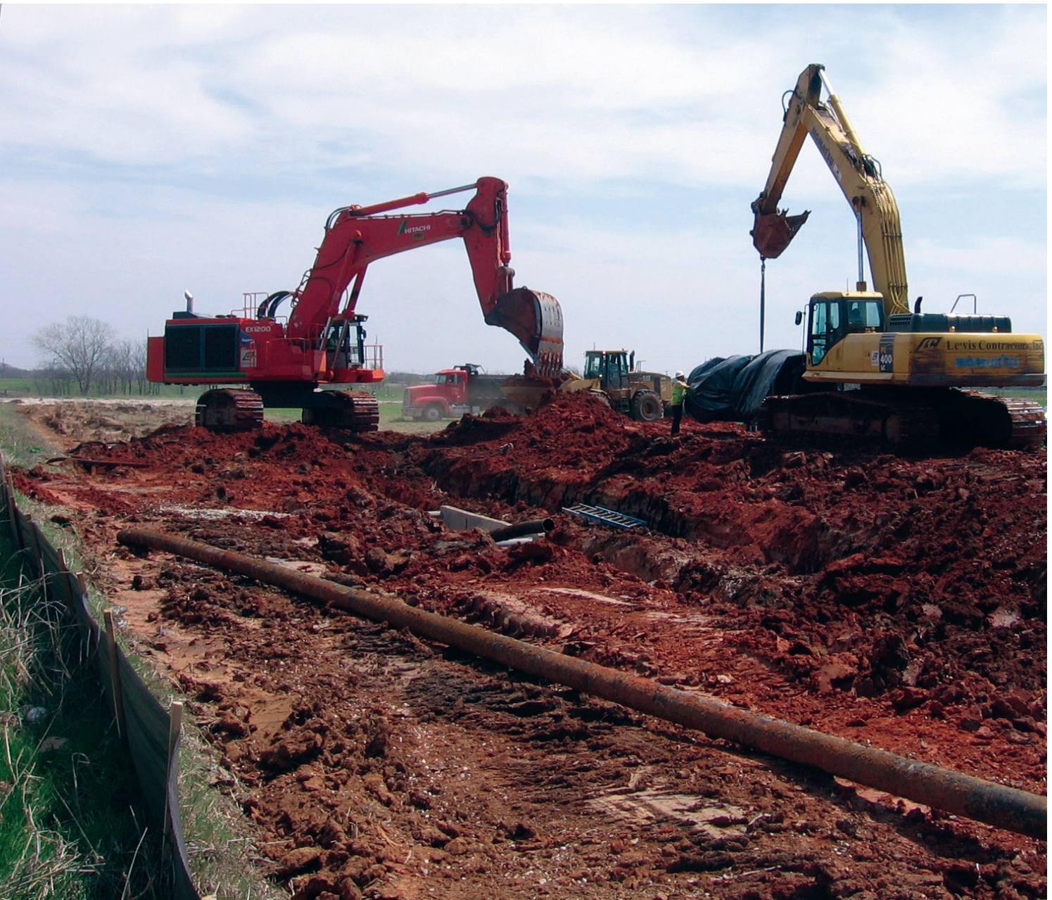
Oklahoma City-Construction of 48" DIP water line.
