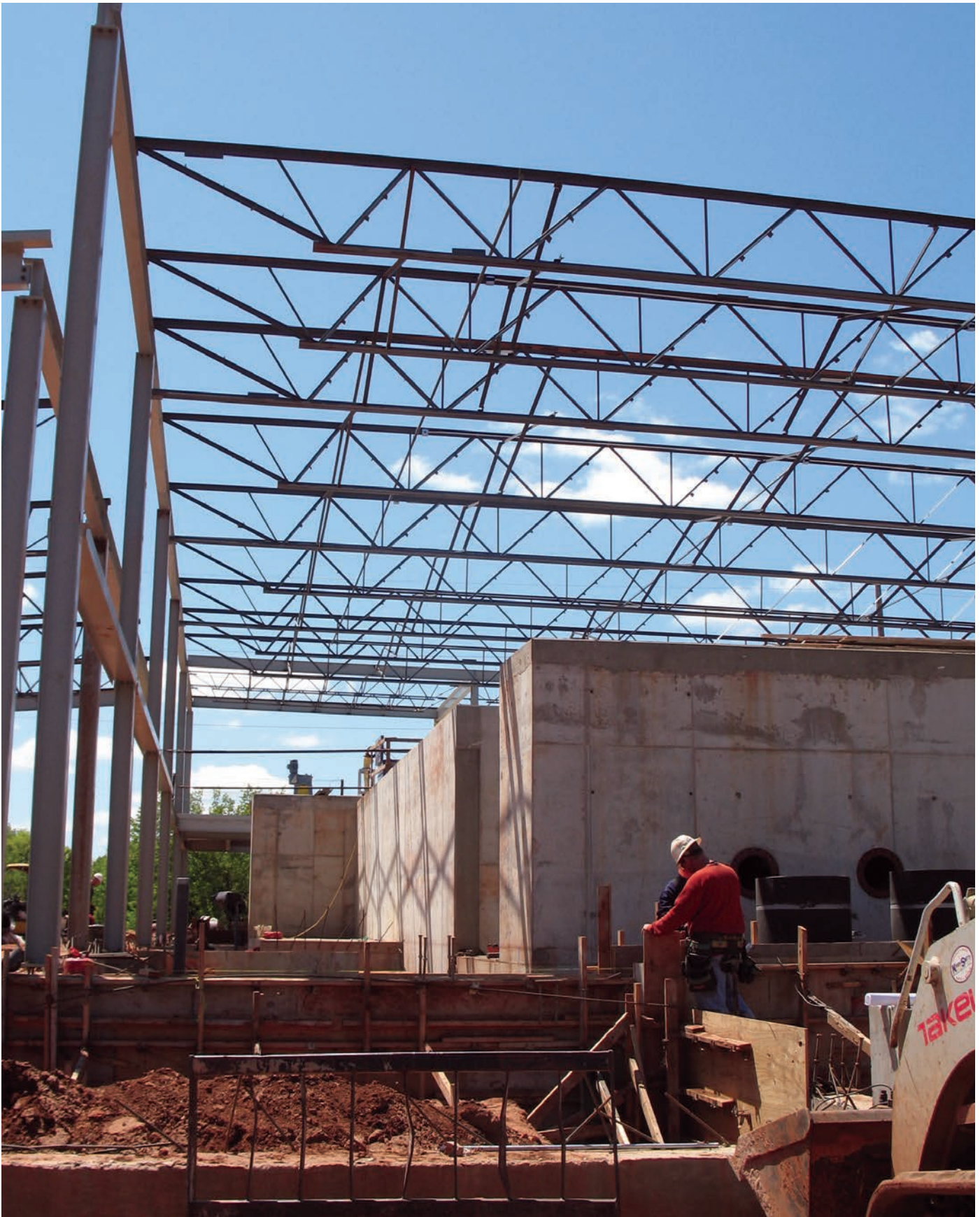
Guthrie-Construction of water treatment plant (process building).
