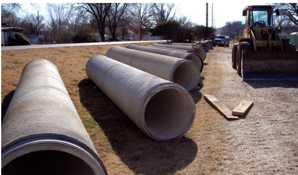
Bartlesville-Construction of Prestressed Concrete Pressure pipe 36" water line.
