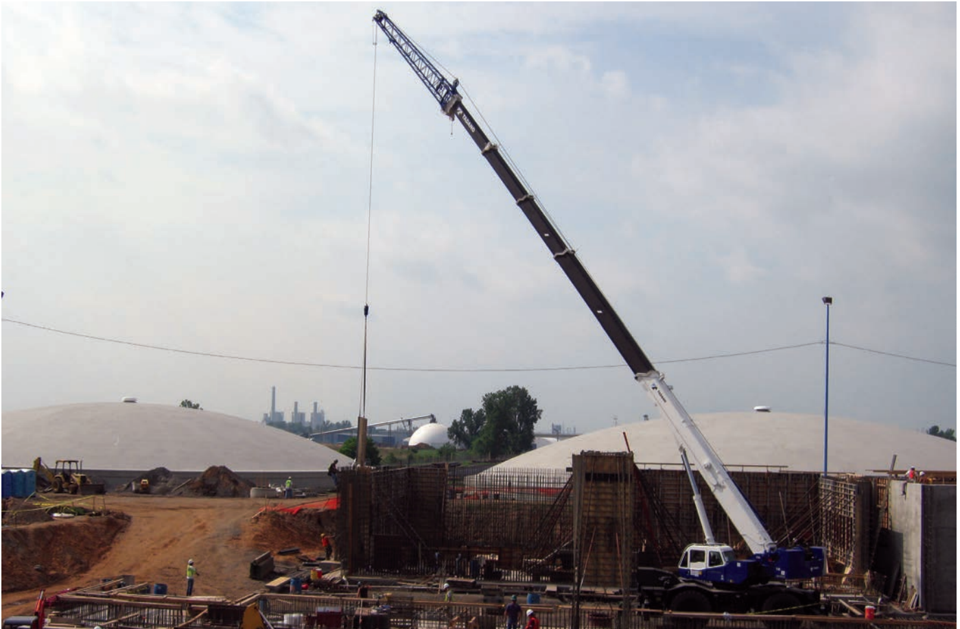
Muskogee-Construction of Water Treatment Plant.
