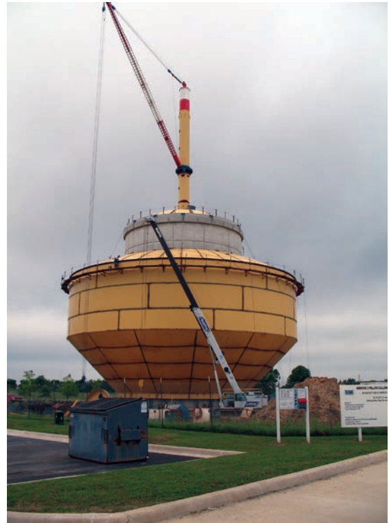
Ardmore -Construction of 2 million gallon elevated storage tank.
