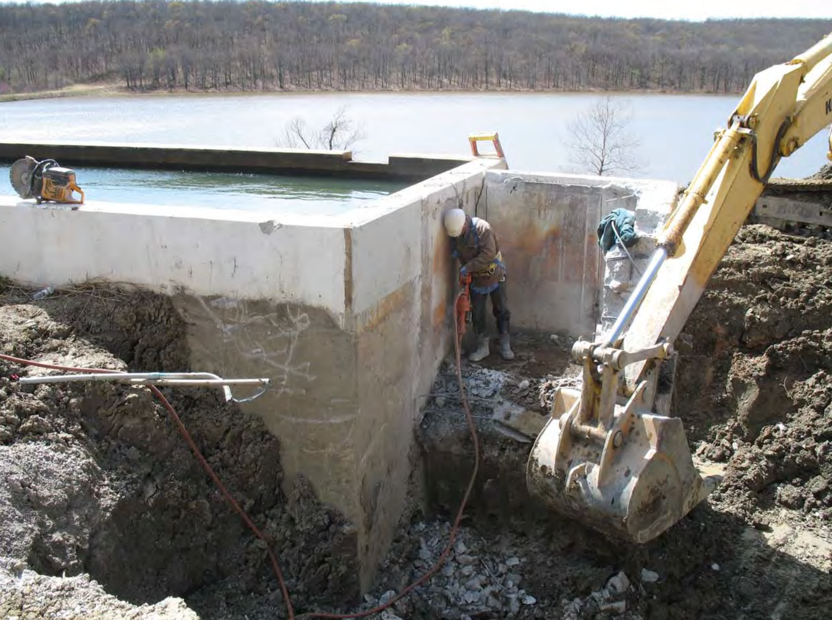
Above: Creek #7 Demolition of the Pre-Sedimentation Basin #2.
