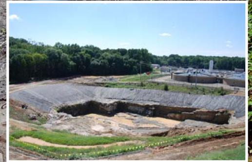
Construction at the Muddy Creek WWTP in Winston-Salem (CS370399-08)
