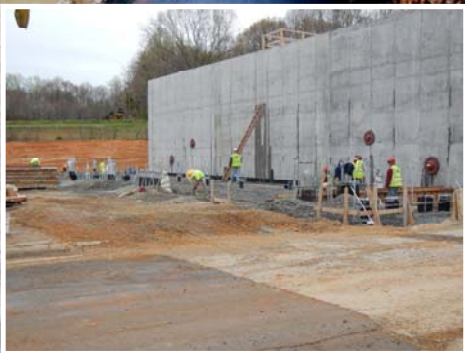
City of Reidsville WWTW Improvements (CS370384-05)
