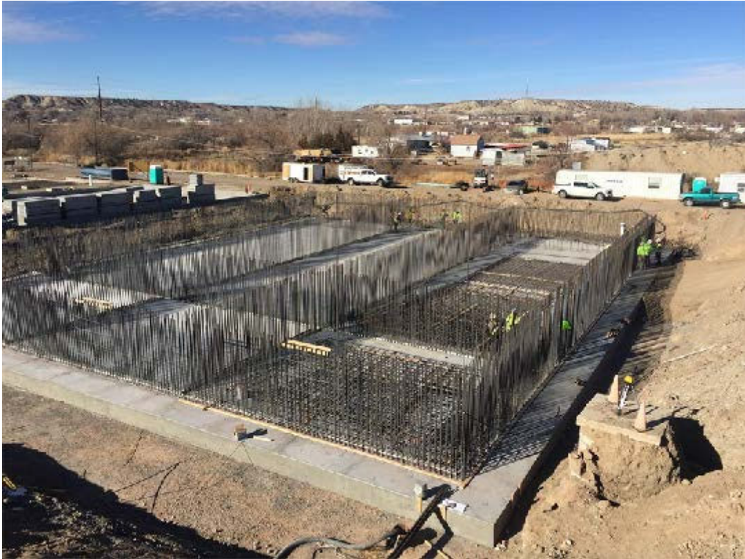
The Town of Bloomfield CWSRF 103 WWTP Construction
