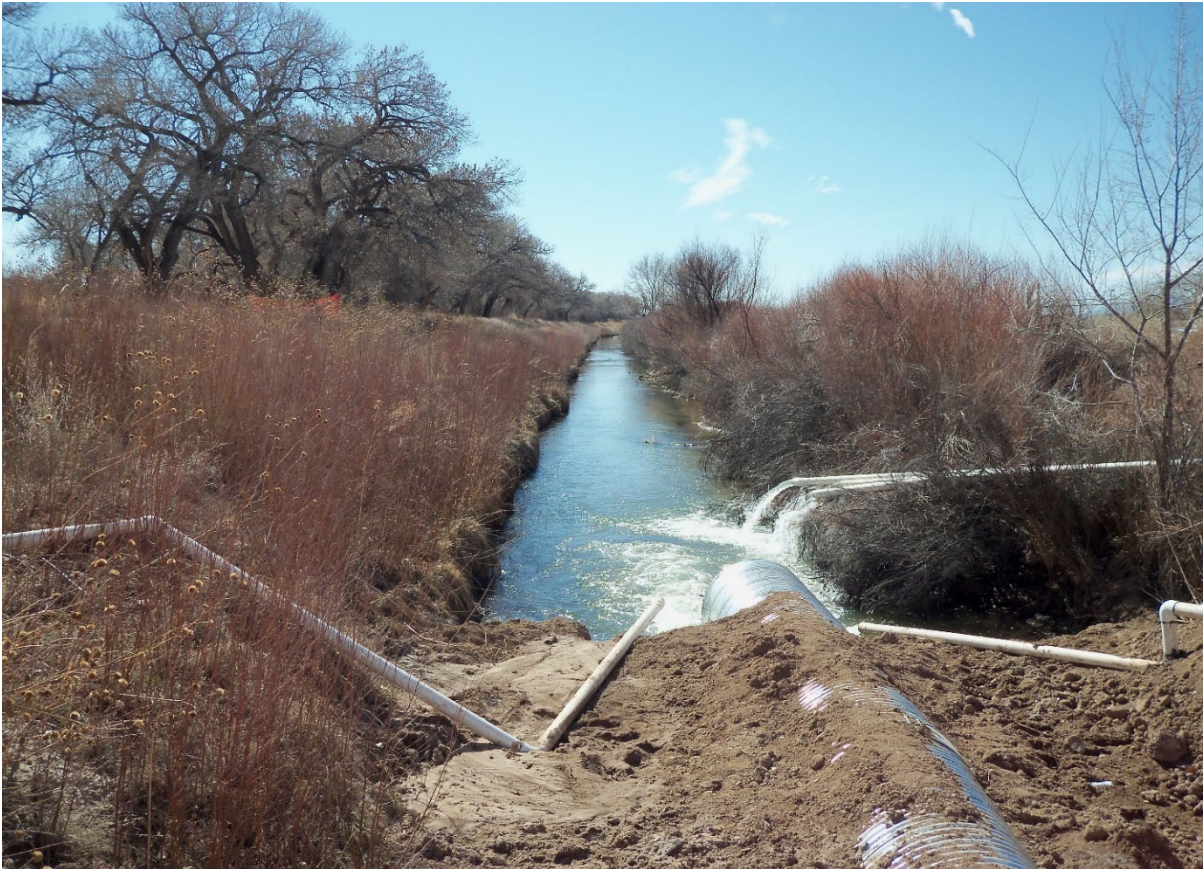
Village of Los Lunas CWSRF 060 Effluent Line Project
