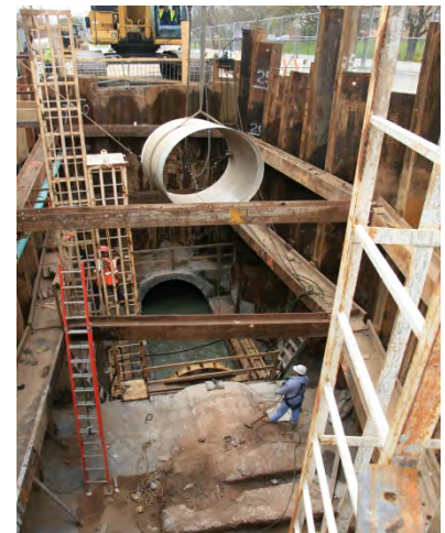
Passaic Valley Sewerage Commission Interceptor Slip Lining
