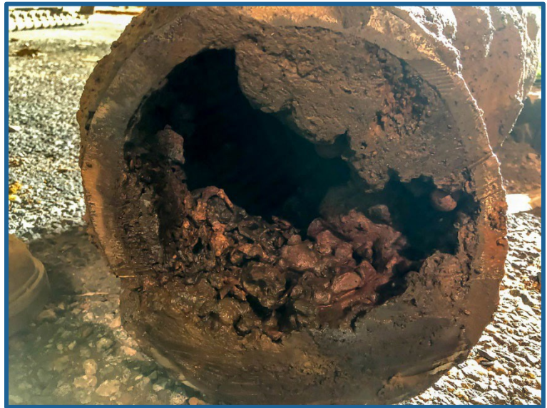
Jersey City MUA Water Main Replacement
