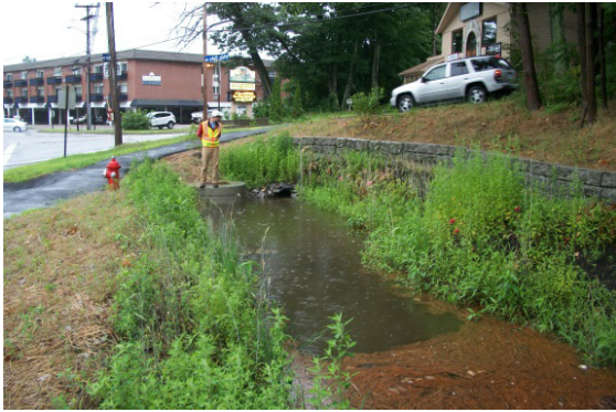
Bio-retention basin to capture stormwater runoff in Laconia.
