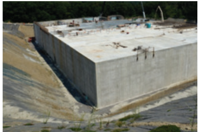
MWRA Spot Pond Storage Facility
