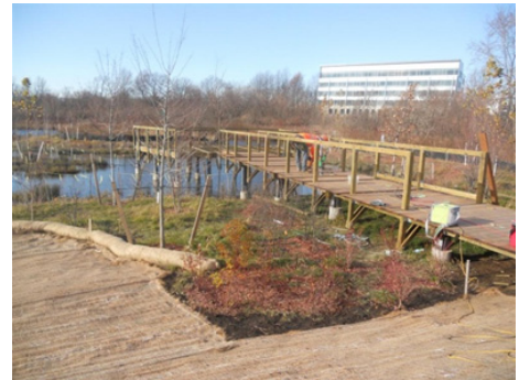
Constructed Wetland and Boardwalk
