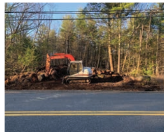
Grubbing and culvert installation.
