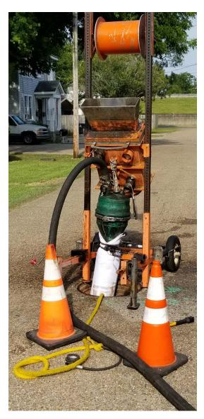
Picture 1: Contractor performing CIPP lining "cooking" process
