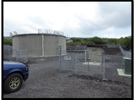
▲ HOVE well site
