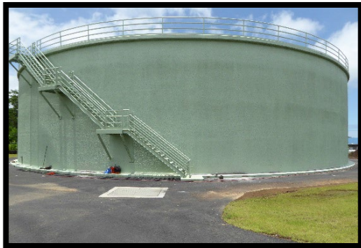
▲ New 2.0 MG tank
