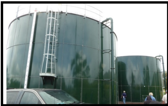
▲ New 228k-gallon steel tanks
