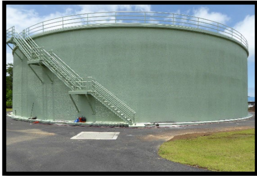
▲ New 2.0 MG tank
