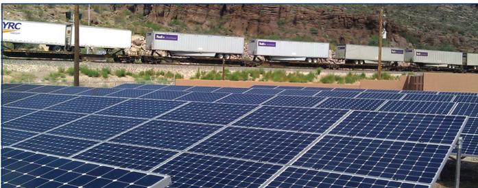
**Kingman** received a WIFA loan in 2012 for construction of their **Downtown Wastewater Treatment Plant (.5MGD)** including a 50 kW-DC solar system. Engineer Phil Alred indicates, "Solar has been a good addition to the plant," meeting 20% of the plant's energy needs and is virtually "plug and play" to maintain. While Kingman had no comparative savings with the new plant, he said WIFA's debt forgiveness helped "solar show a good ROI."
